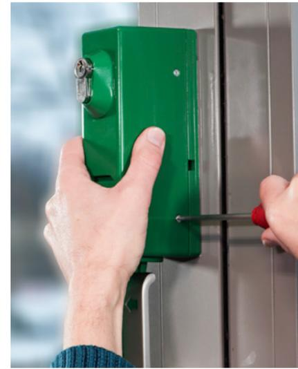
**It is essential to ensure that the release path of the window handle is guaranteed up to its end stop. The GfS Flügelwächter® and its installation aids must completely release the actuation path of the window handle after triggering.**
