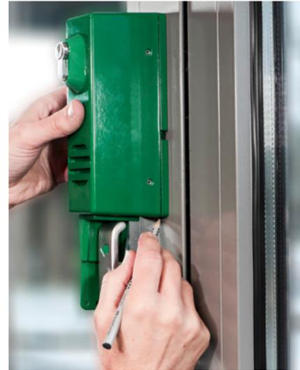
1a. If you use the mounting plate for fire doors: Clean the frame thoroughly by removing grease and dust. Remove the protective foil from the adhesive surface. Press the mounting plate with the sticky side against the frame for approx. 10 – 15 seconds as marked before.
